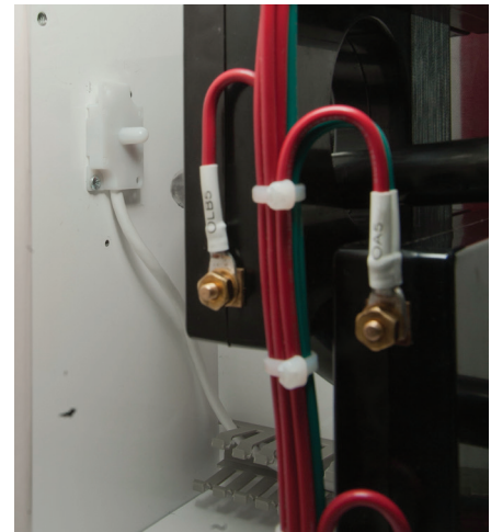
Examples of appropriate point sensor installation.
